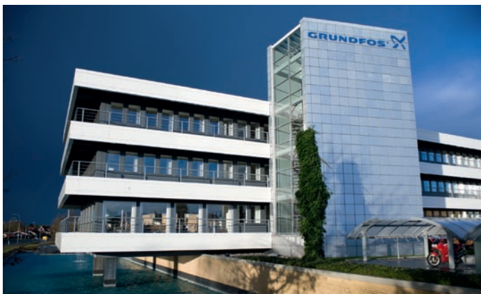
Imposant: Das Grundfos-Headquarter in Bjerringbro/Dänemark.
